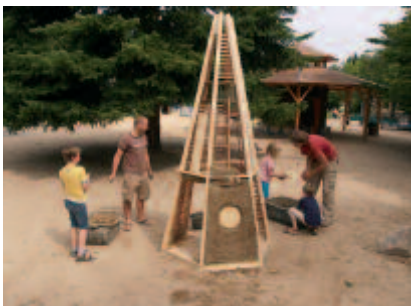
Figure 2. Constructing an earthen tipi (Photo R. Warzecha 2005-2008).
